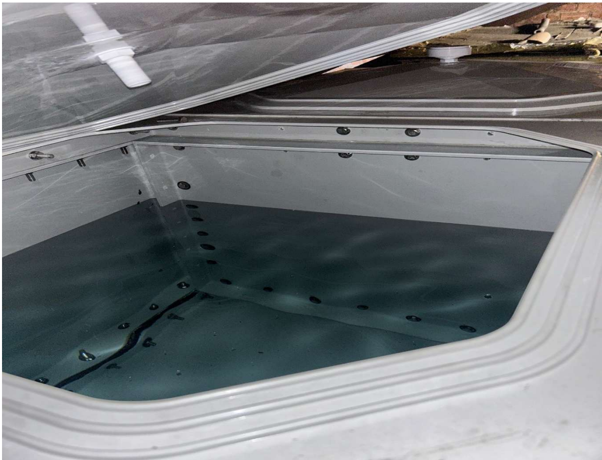
NEW COLD WATER STORAGE TANK VIEWED THROUGH TOP ACCESS LID
